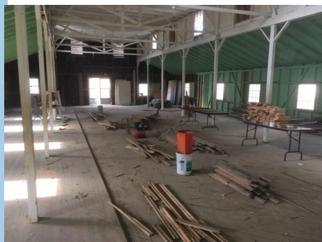
Interior floor nearly removed
