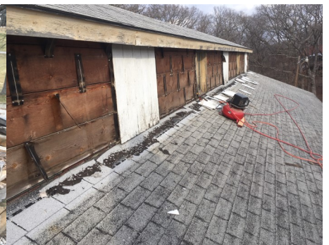
Removing the upper siding
